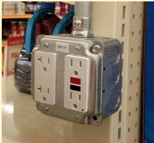
wires from the panel to the outlet due to the height of the ceilings. The locations for the coolers were previously mapped out by their corporate, so the techs had to be sure to run the circuit to the precise location.
